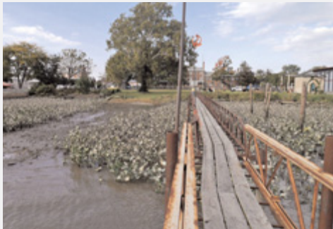
Ramp on left and dock leading to Lazaretto
