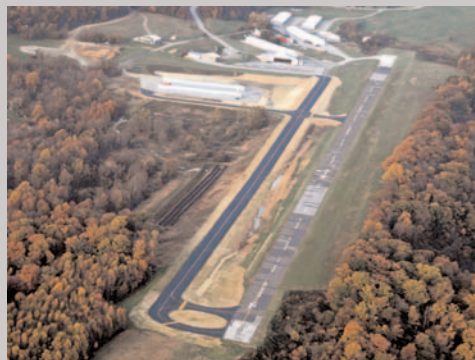
New taxiway at New Garden Airfield
