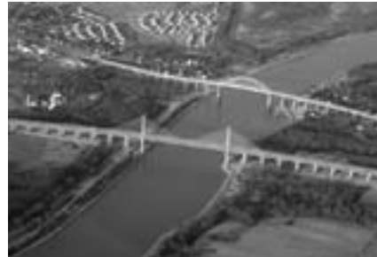
Cable-Stay Bridge, C&D Canal
