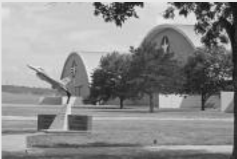
The Museum is housed in 3 large buildings on the west side of the old Wright Air Force Base.
