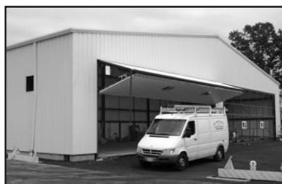
New equipment building at Wings
