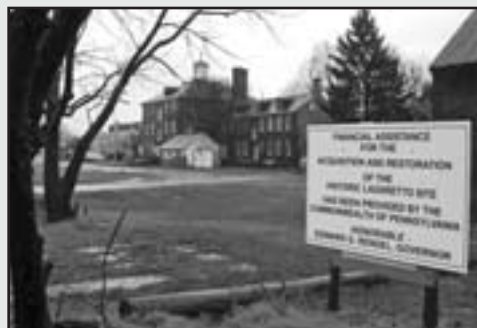
Historic Lazaretto House under restoration
